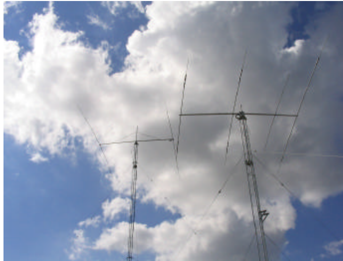
Above: Part of the W8EDU Antenna Farm
